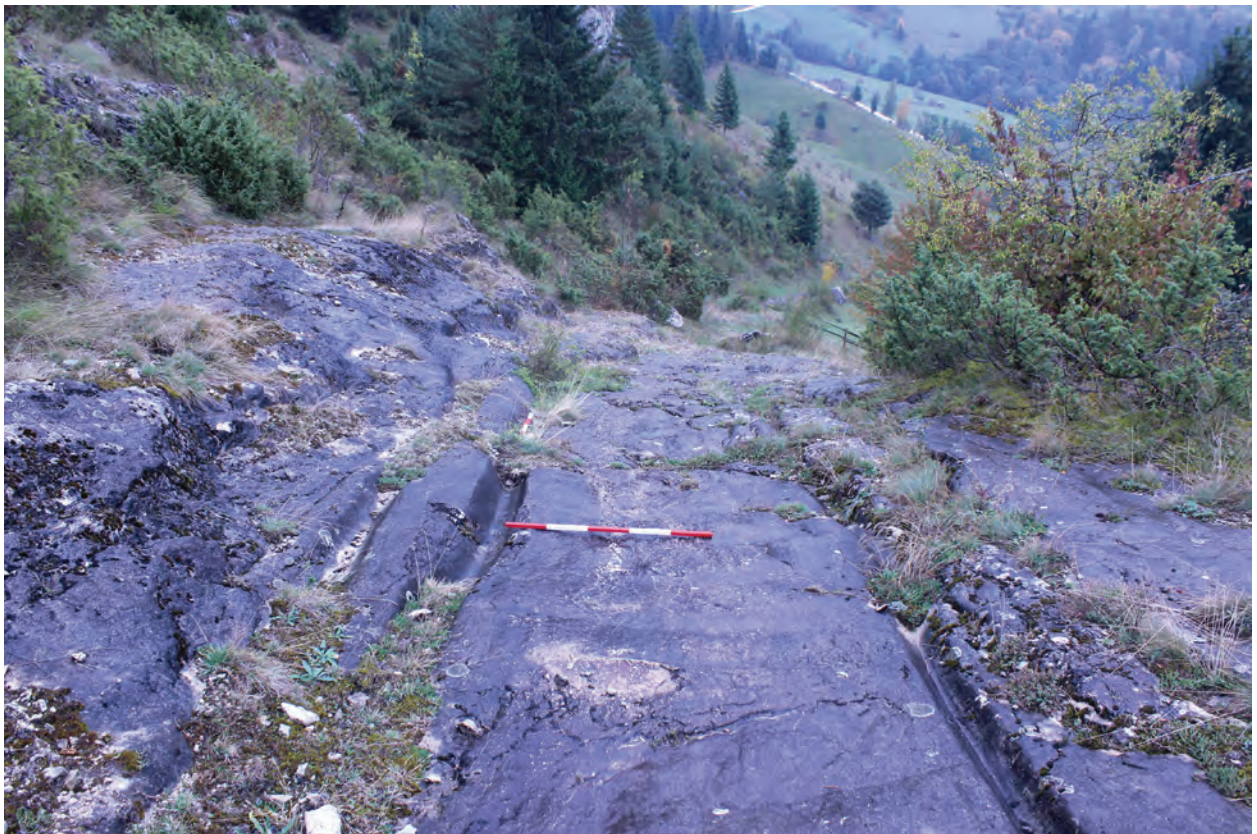
Fig. 8. The trace of the road running along the western side of the castle (photo taken by the author).
